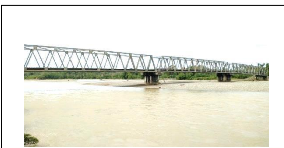
Gambar 1. Eksisting jembatan Alue Buloh
