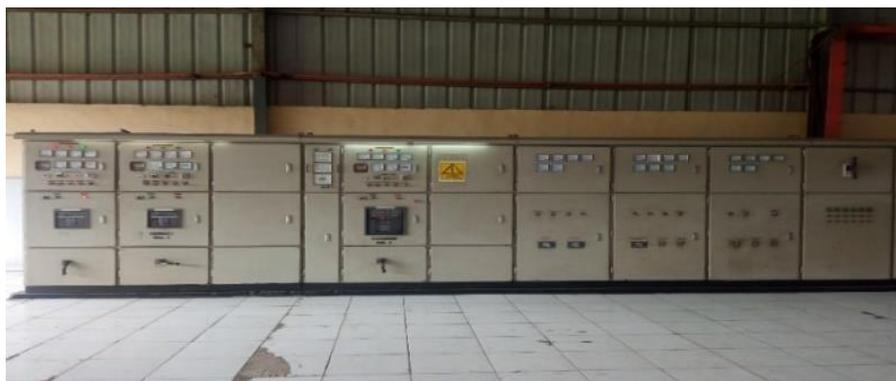
Gambar 3. Main Switch Distribution Board (panel)
