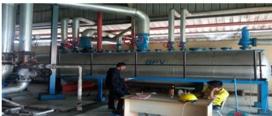
Gambar 4. Back Pressure Vassel (BPV)
