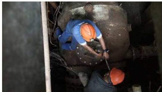
Gambar 10. Pembukaan Manhole Debris Filter
