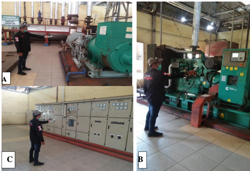
Gambar. 2 Pengukuran Pengujian Kebisingan A;Turbin, B;Genset, C; main switch distribution board (panel)
